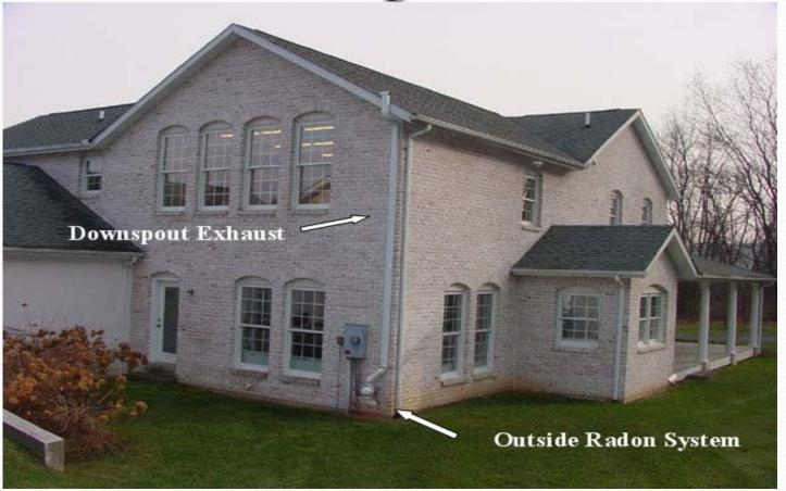
Most mitigation systems can be designed to blend into the natural structure and utilities of the home
